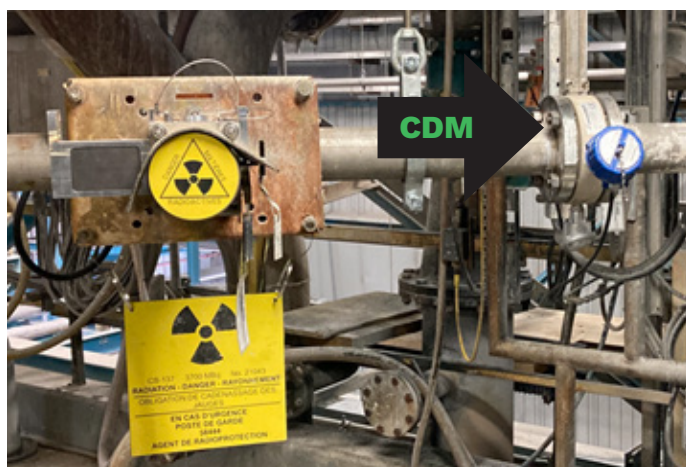
The CDM installed in the same line as where the radiation-based density meter is measuring density
