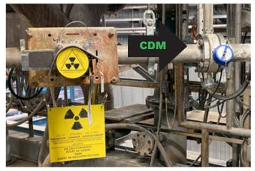
The CDM installed in the same line as to where the radiationbased density meter is measuring density
